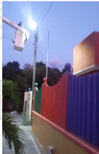
CHEMUYIL, SE REHABILITAN REFLECTORES (TIPO AM1,000W Y BALASTROS AM1,000W).
