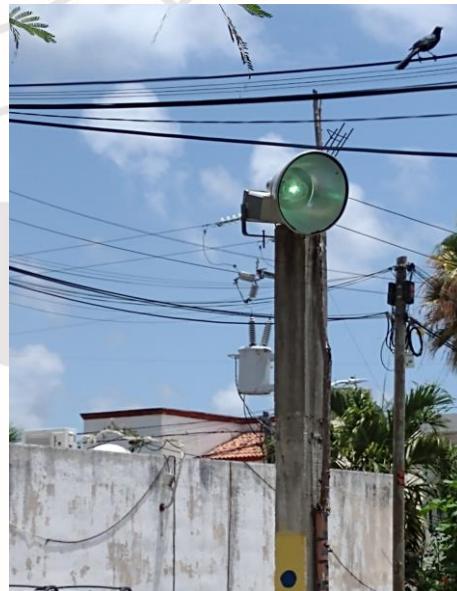
VILLAS TULUM, SE REHABILITAN 2 REFLECTORES (TIPO AM1,000W Y BALASTROS AM1,000W)
