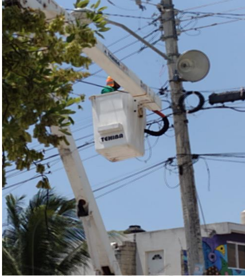
AKUMAL, SE REHABILITAN REFLECTOR (TIPO AM1,000W Y BALASTROS AM1,000W).
