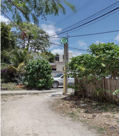
VILLAS TULUM, C. CHEMUYIL / C. 2 BIS, SE REHABILITAN REFLECTORES (TIPO AM1,000W Y BALASTROS AM1,000W)
