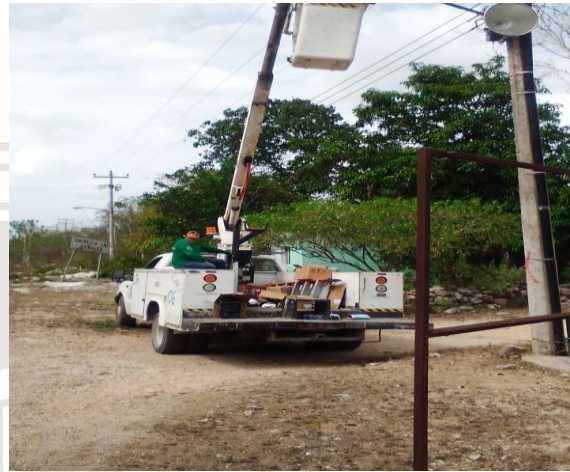
YALCHEN , SE REHABILITAN REFLECTORES (TIPO AM1,000W Y BALASTROS AM1,000W).
