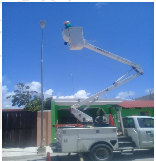
TUBEN KA, C. 30 Y AV. 18, SE REHABILITA LAMPARA LED 100 WATTS.
